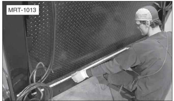
4. Measure and determine the centerline of the truck's rear sill. Mark this point.
