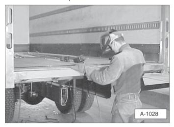
Lift and center the liftgate on the truck's rear sill.
